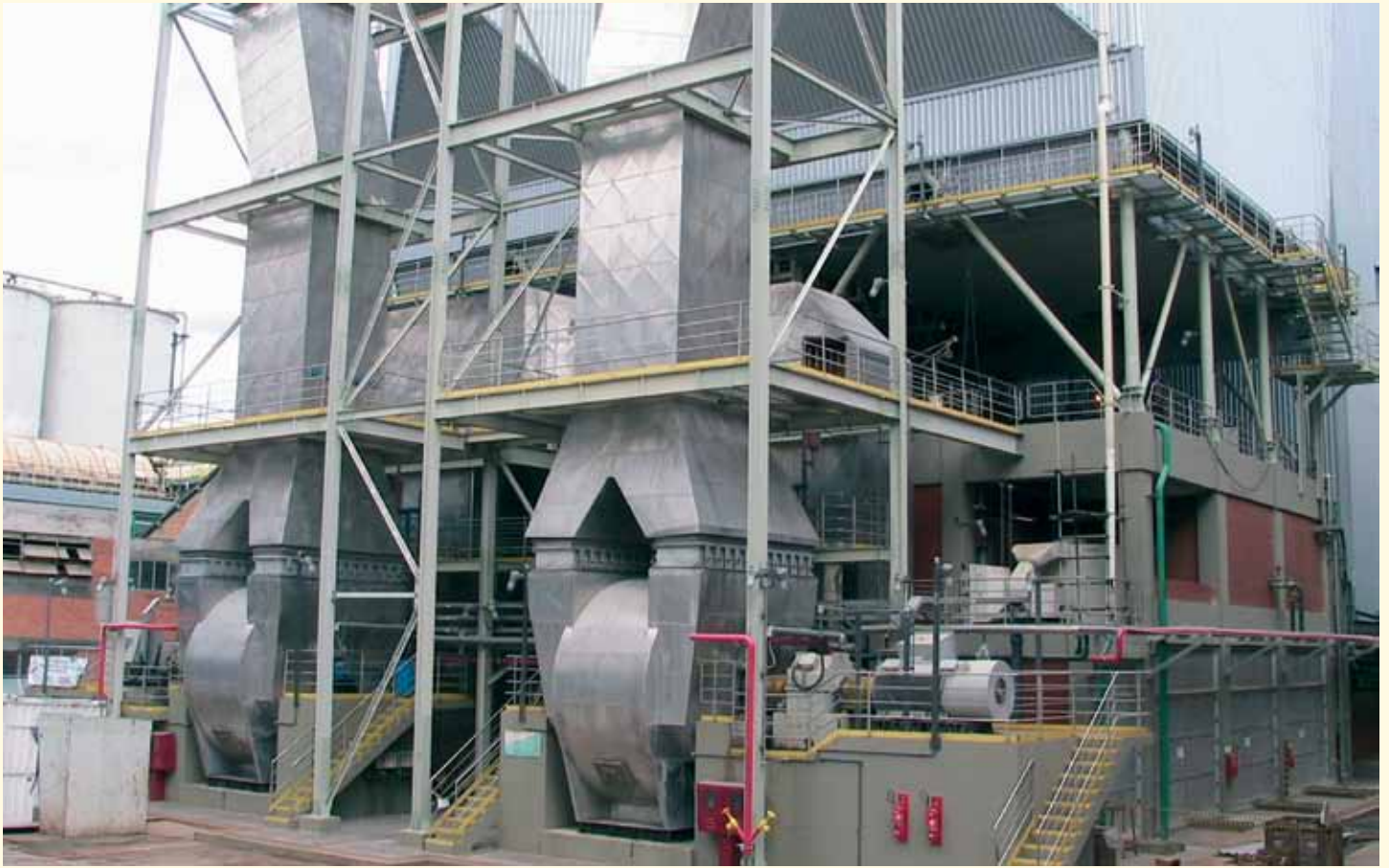
2xD34 KSL, 2000 kW - 1200 rpm, Fan drive (Brazil)
