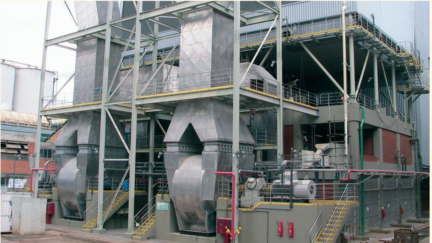
2xD34 KSL, 2000 kW (2682 hp)- 1200 rpm, Fan drive (Brazil)
