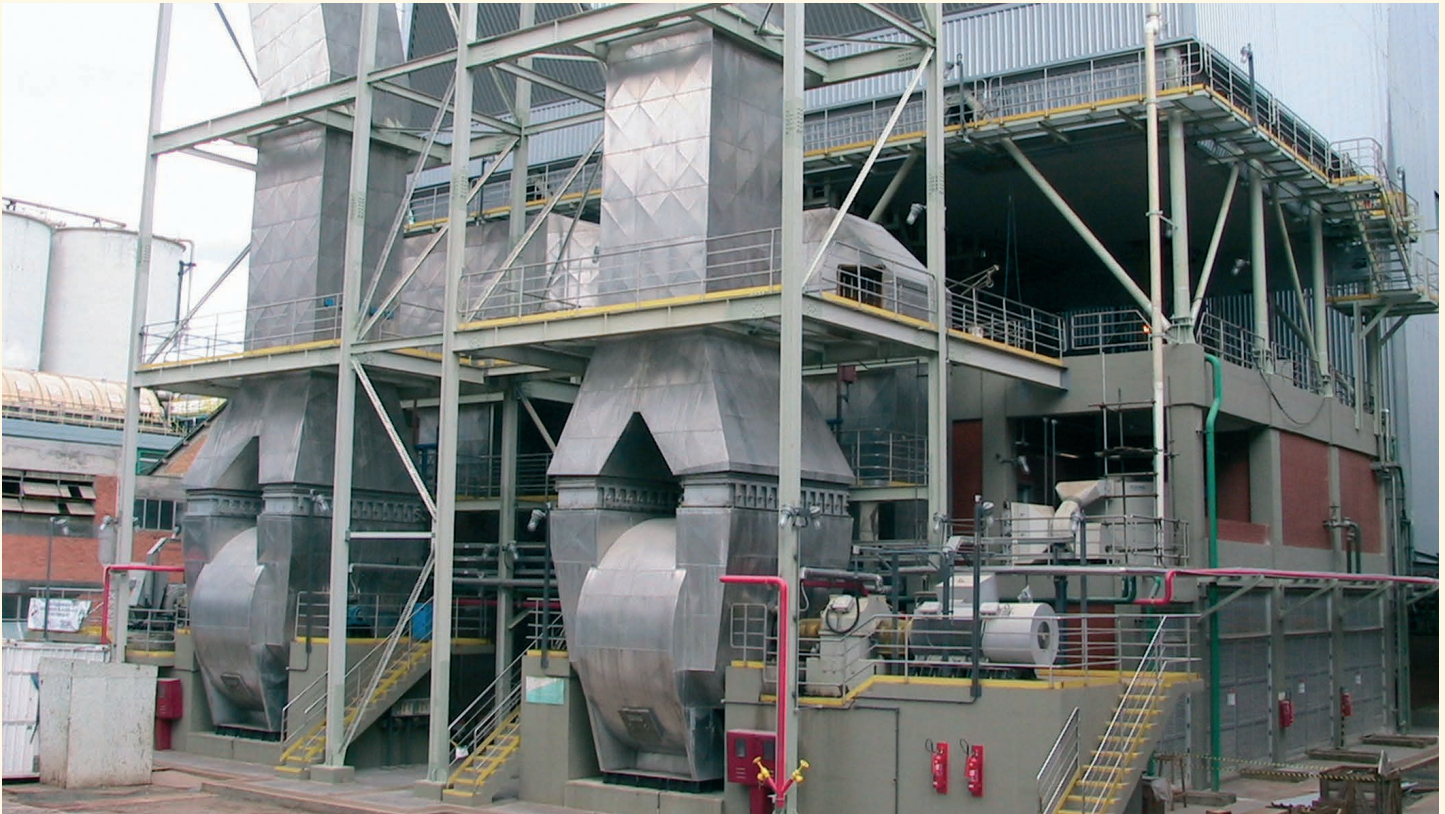
2x34 KSL, 2000 kW (2682 hp)- 1200 rpm, Fan drive (Brazil)
